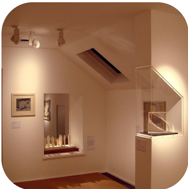
Lighting before LED replacement showing ERCO halogen lamps located in fixed singlets.
